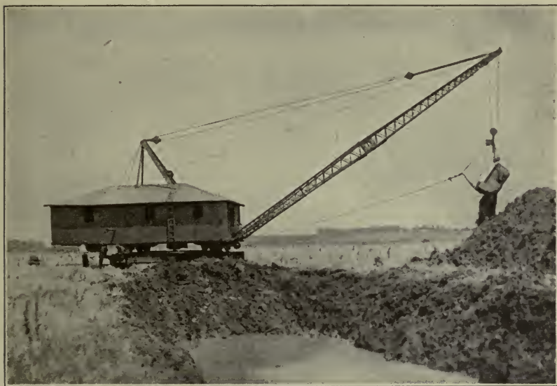
Fig. 31. Revolving Excavator on Caterpillar Tractor Operating on Drainage Work
